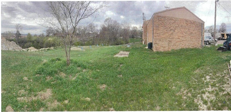
EAST SIDE OF WATER PLANT (LOOKING WEST)
