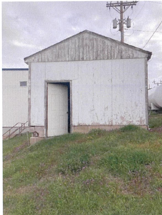
BACK OF GARAGE
