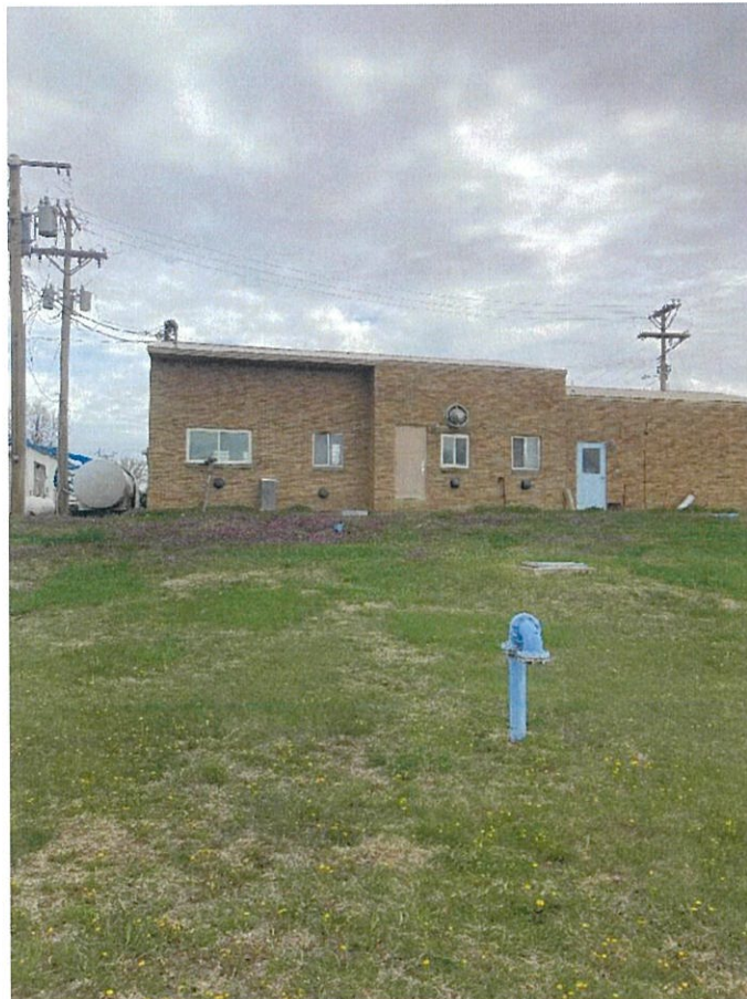
BACK OF WATER PLANT (LOOKING NORTH)
